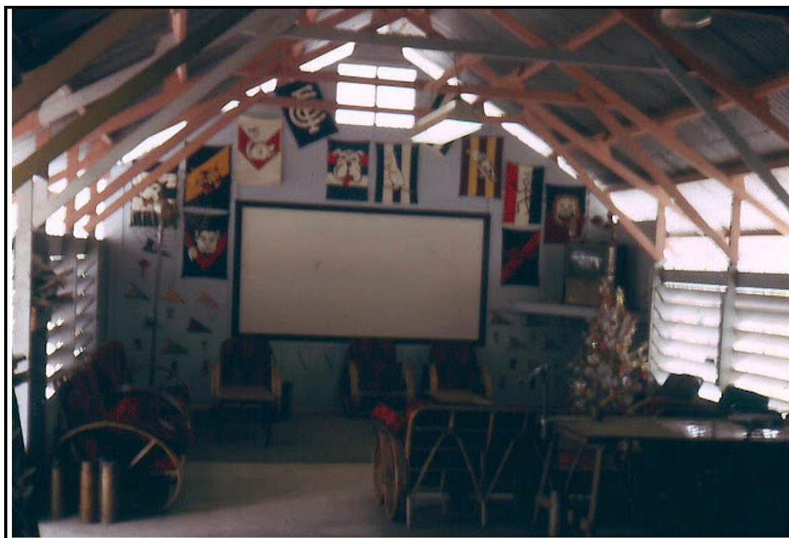
Figure 365: Club interior completed
