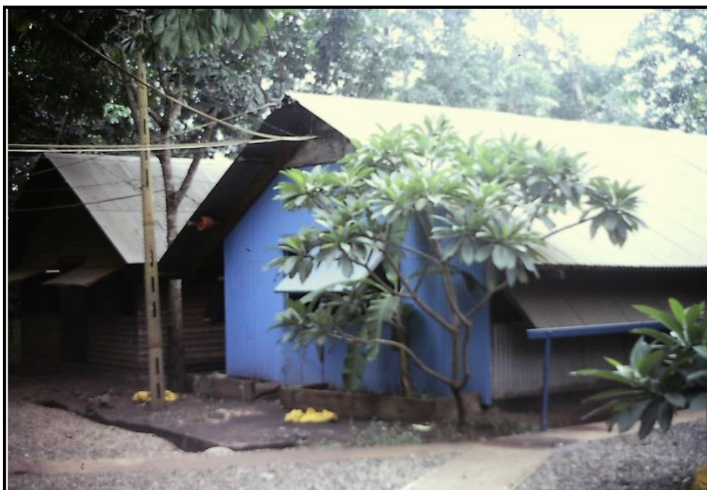
Figure 659: Set Room/ARDF Building
