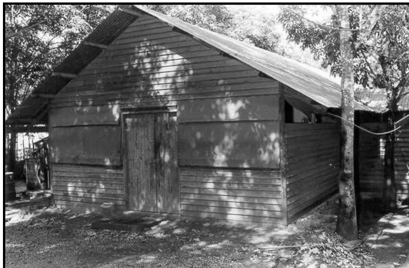
Figure 248: Intelligence/Processing, Stores and Canteen Building
