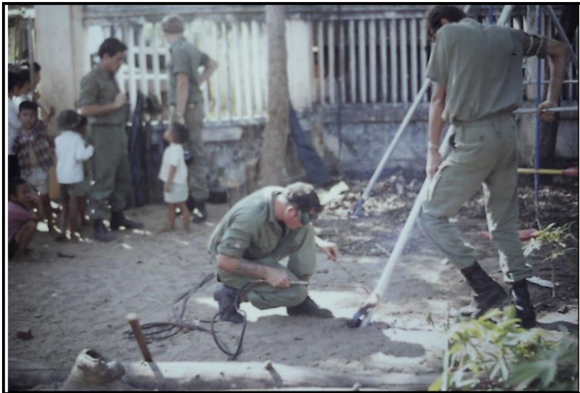
Figure 702: Peter Weir-Smith and Bob Watson erecting the playgym
