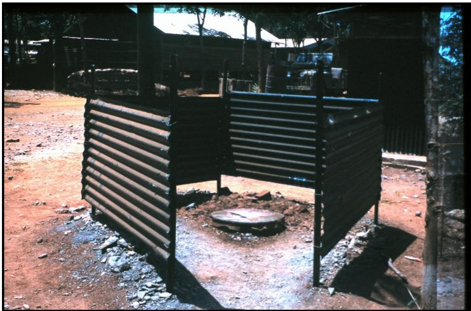
Figure 321: New urinal under construction
