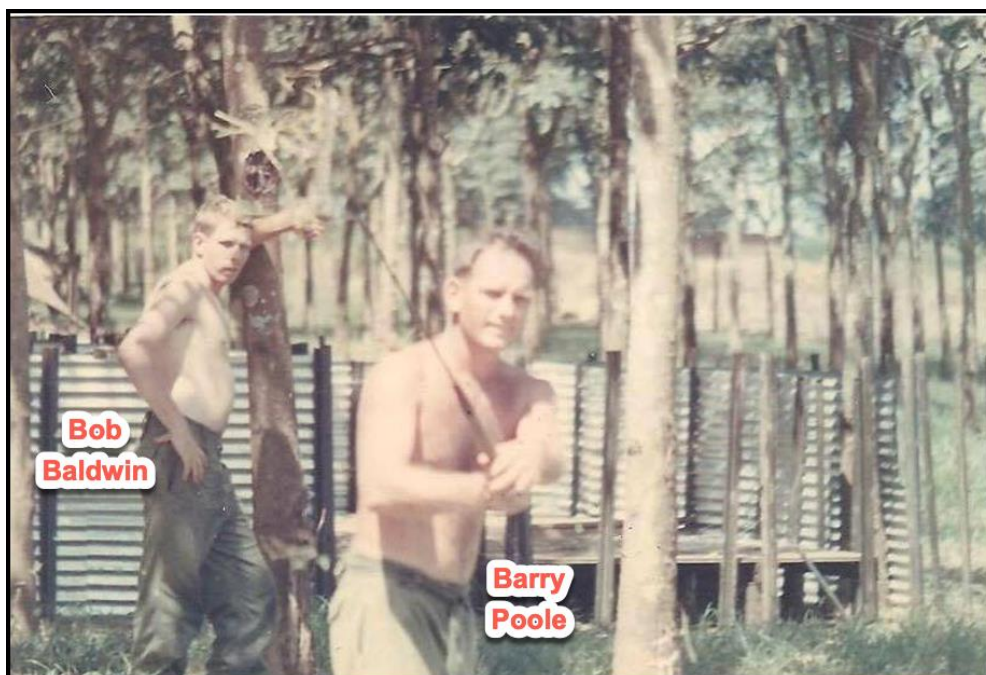
Figure 371: Hard at work during the re-construction
