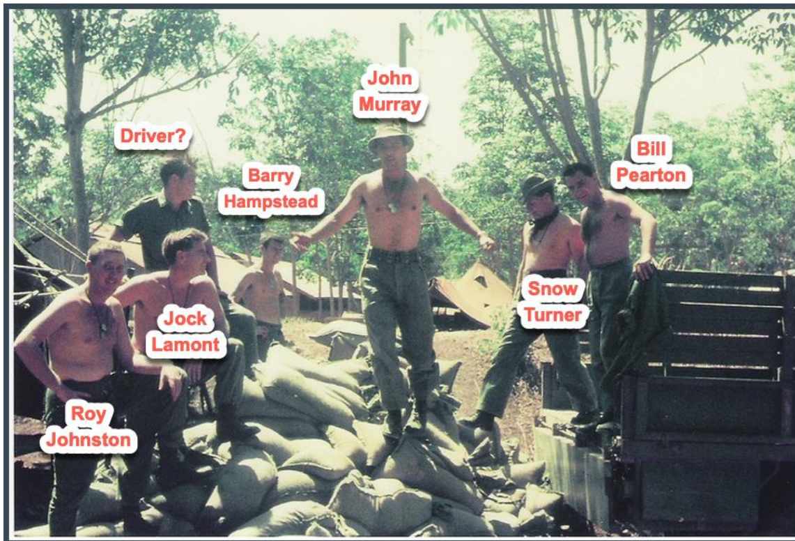
Figure 202: Sandbag filling work party
