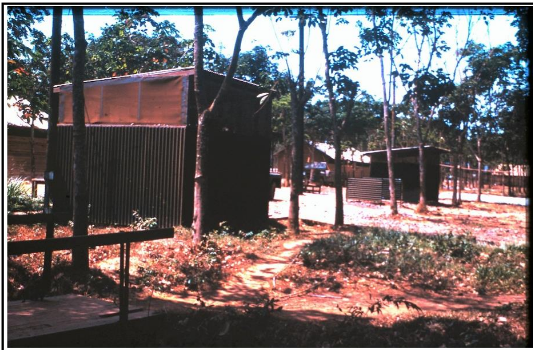
Figure 319: New Shower and Toilet Blocks
