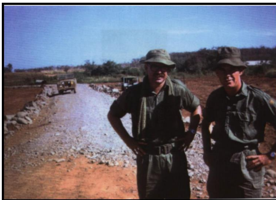
Figure 289: John Peters and Bob (Sadie) Lean 609 at the site
