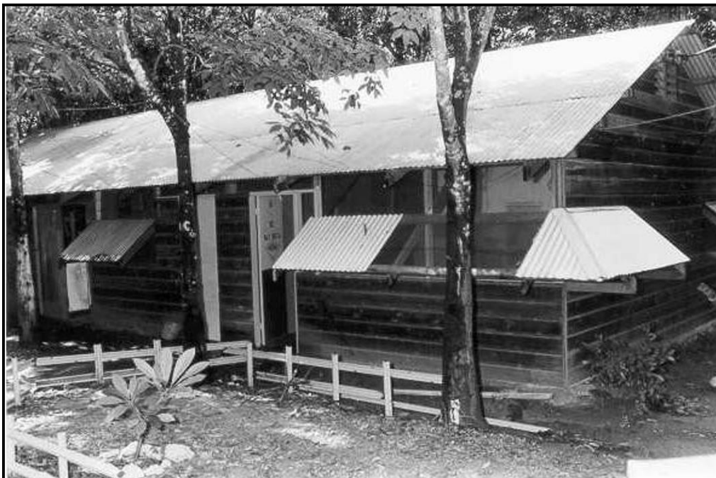
Figure 363: Completed New Building
